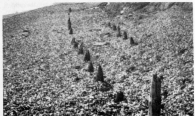
Remains of piles used to support the railway on the beach section, looking west towards Sidmouth. The two lines of piles are 5ft apart: in each line piles are set at 4ft 6in intervals
